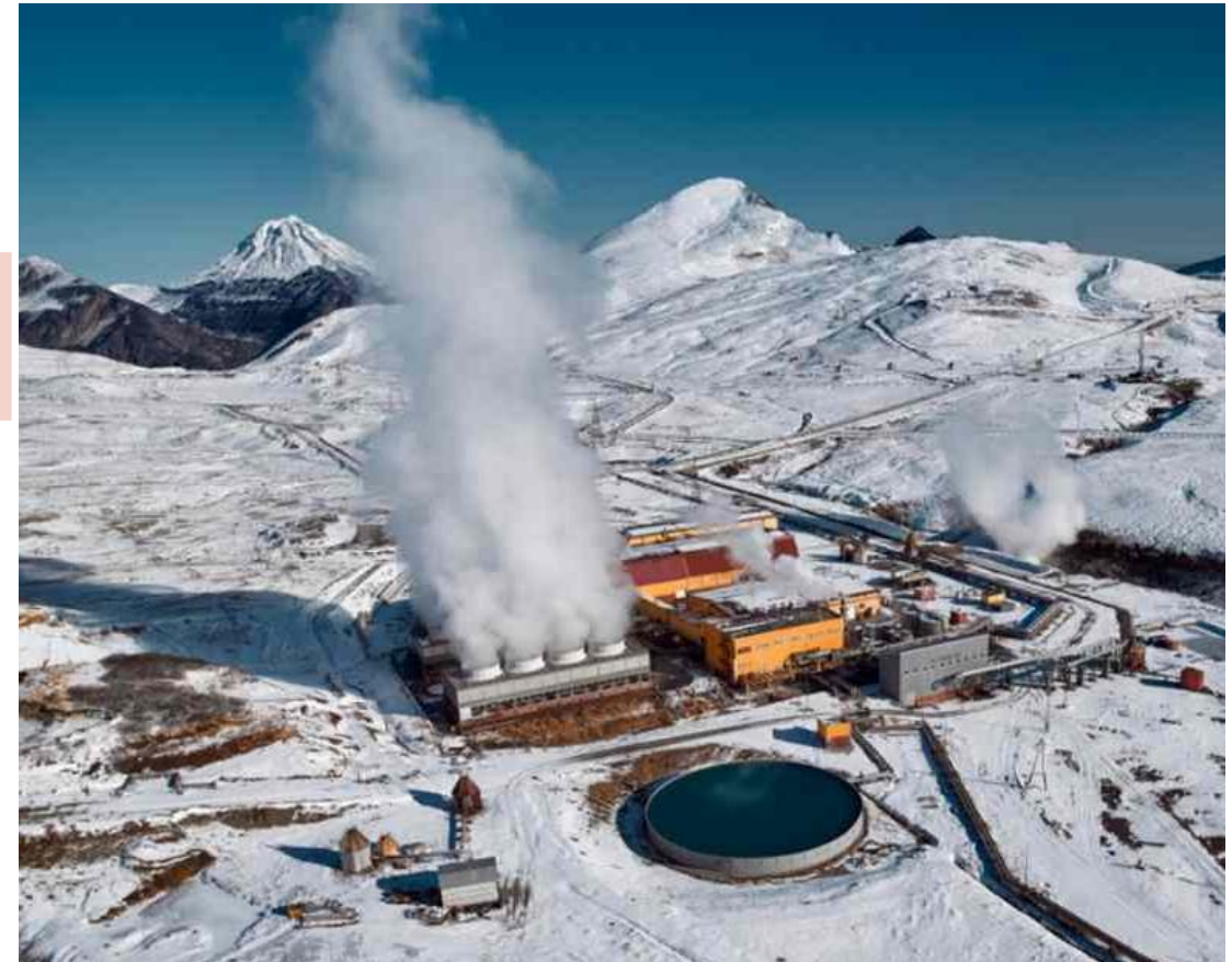
Hydrothermal geothermal power plant in Kamchatka, Russia
